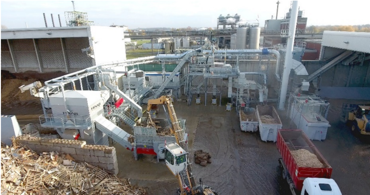
HAAS waste wood processing plant in Cologne-Niehl
